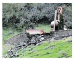
the contractor failed to conduct a proper soil analysis, and that both the base and the retaining wall were inadequately designed and constructed. The IE estimated the cost to
