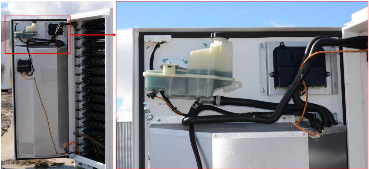
Figure 9 Powerpack thermal door (left) and close up of the refrigerant (right)
