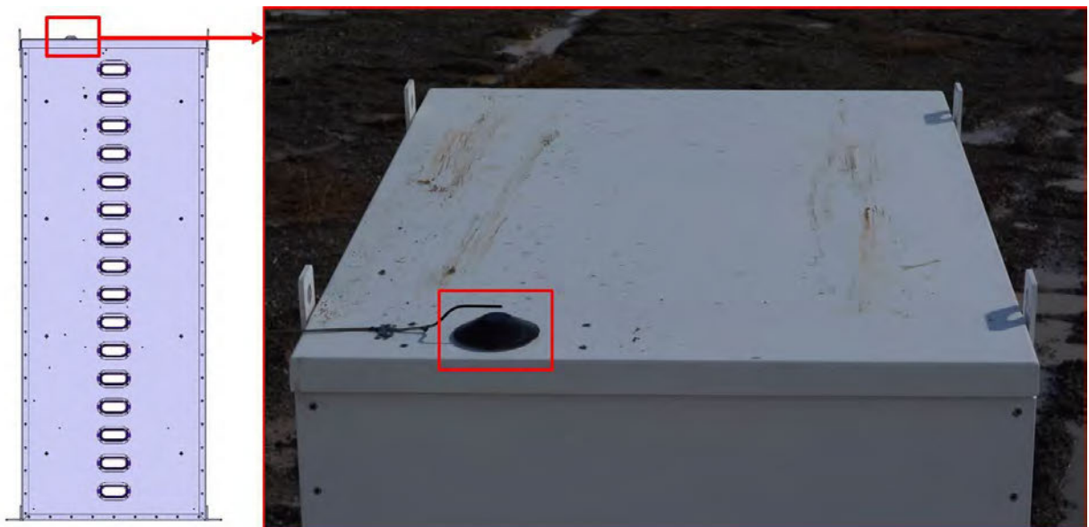
Figure 10 Illustration of the Powerpack exhaust vent (left) and an image of the vent at the top of the Powerpack (right)
